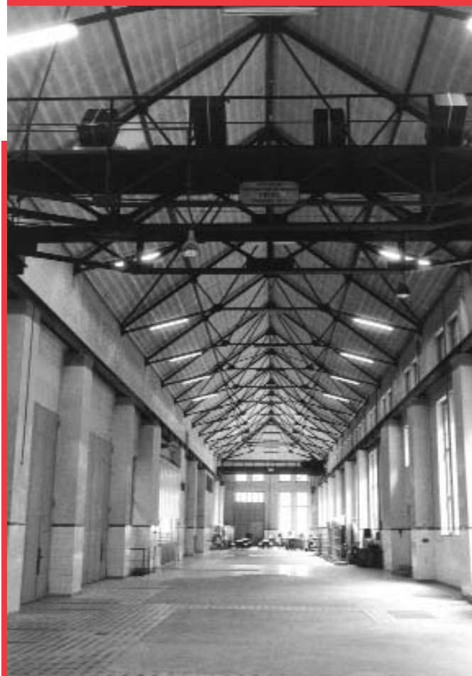
OW: Turbine Giswil
